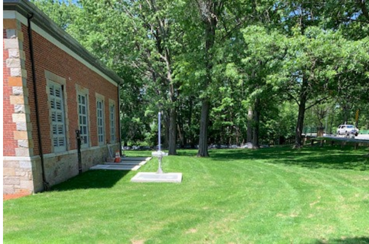
View of the Grounds at Alewife Brook Pump Station
