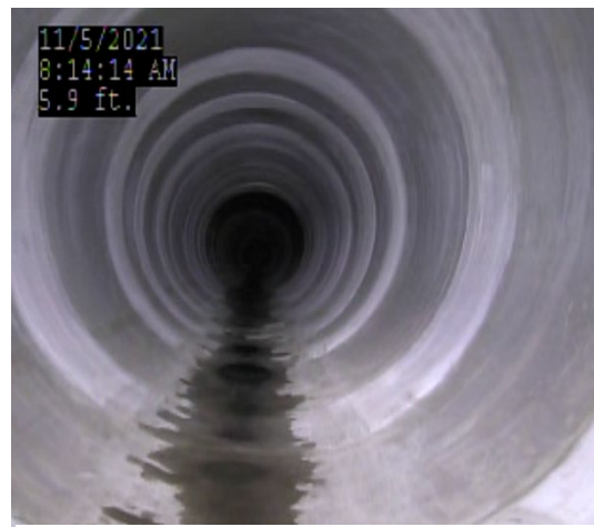
WASM 3 Cleaned and Lined Piping
